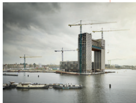
Four Liebherr cranes in Amsterdam
