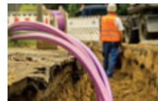
◀ 12 to 14 bar: Cable blowing and drilling
