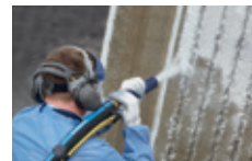
◀ 8.6 to 10 bar: Abrasive blasting
