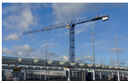
Loads up to 13.2 tonnes will be handled by the 50 tonne capacity crane
